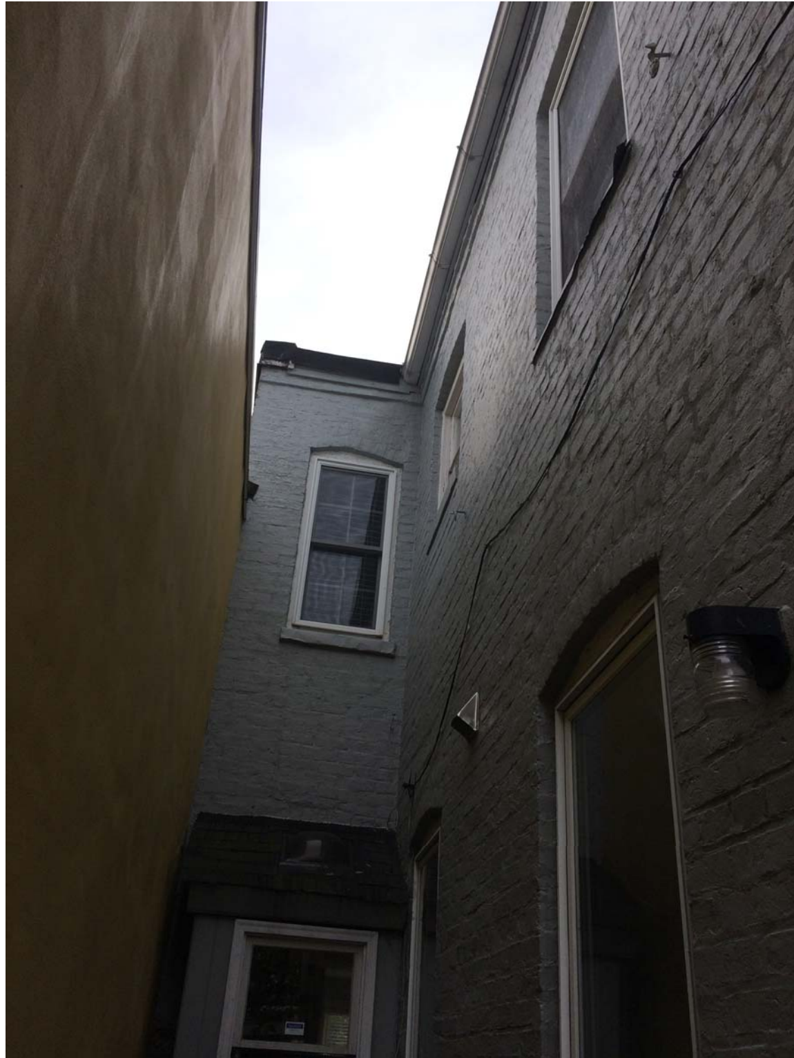
VIEW OF EXISTING DOGLEG @ 656 INDEPENDENCE AVENUE SE
