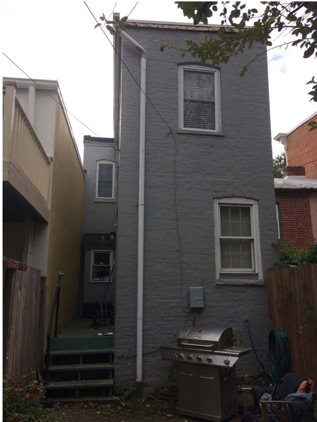
EXISTING REAR FAÇADE
