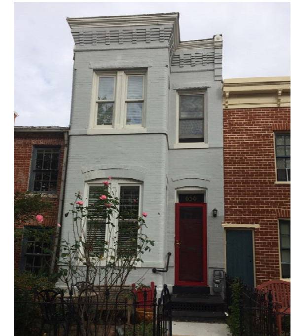
VIEW FROM INDEPENDENCE AVENUE SE
