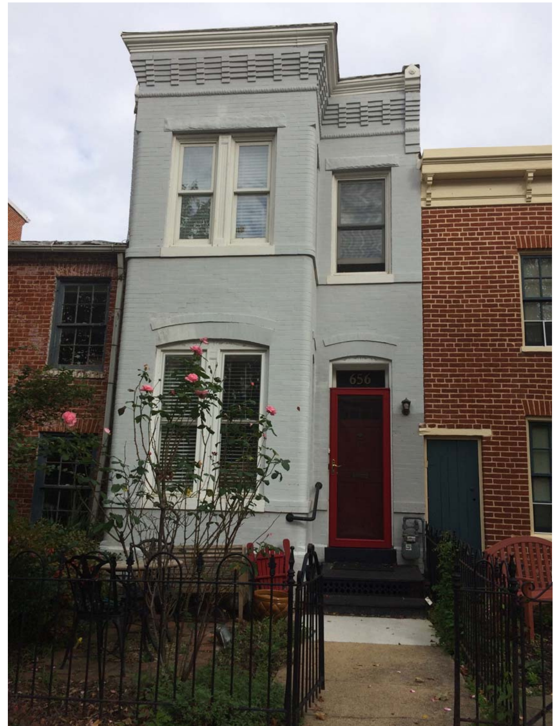
EXISTING FRONT FAÇADE
